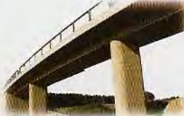
a concrete bridge
